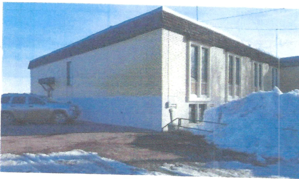
View: West elevation of the site building, looking northeast
