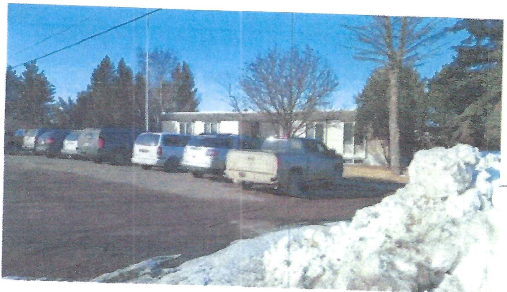
View: East elevation of the site building, looking southwest
