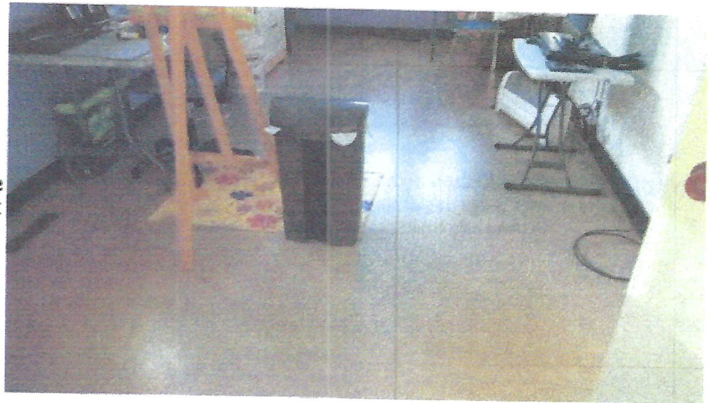
View: Typical tile located in the basement
