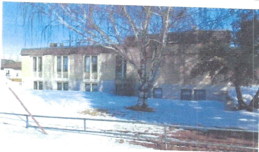
View: South elevation of the site building, looking north
