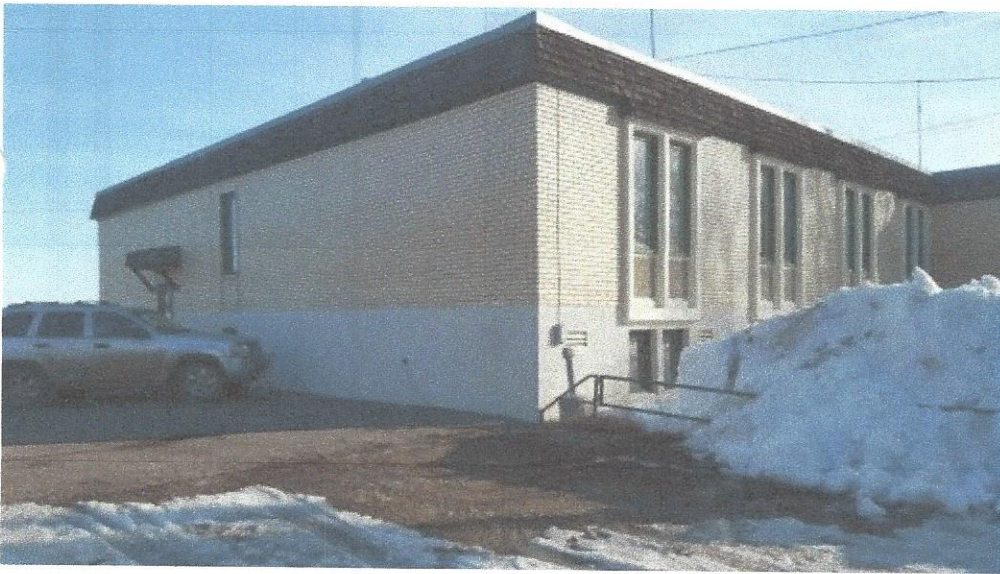
View: West elevation of the site building, looking northeast
