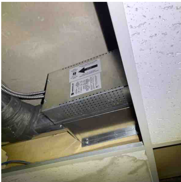
8.1.2 Some limited and operational electrical baseboard heating. In duct work heat system for the future potential suite was operational
