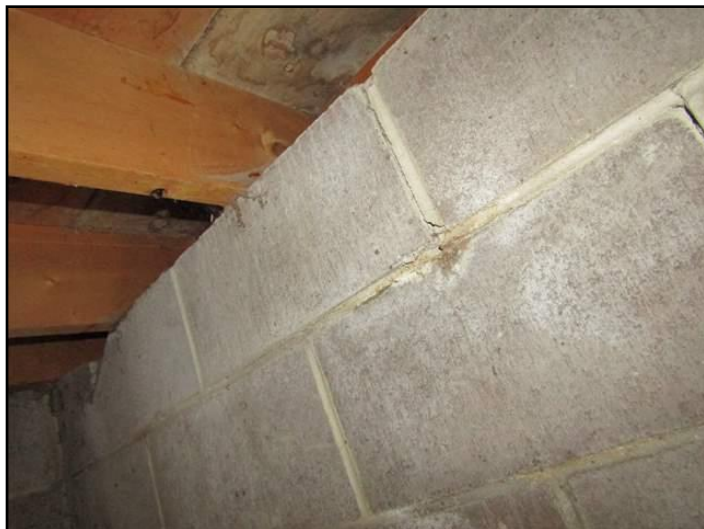
Step crack
