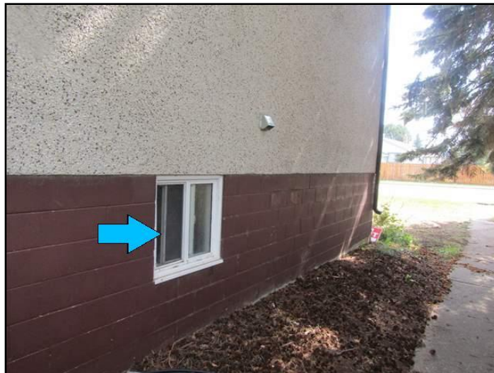
Unit 2 bathroom window
