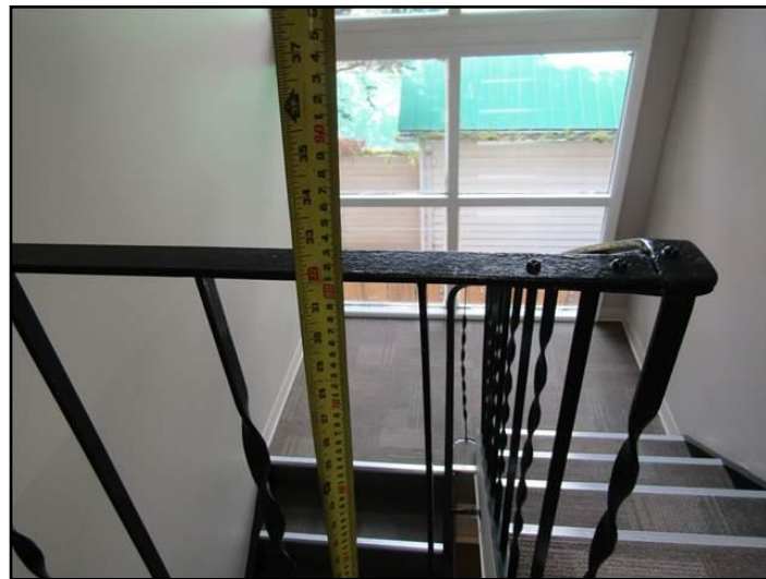
32" stairwell handrails
