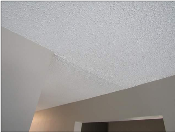
Settlement cracks
