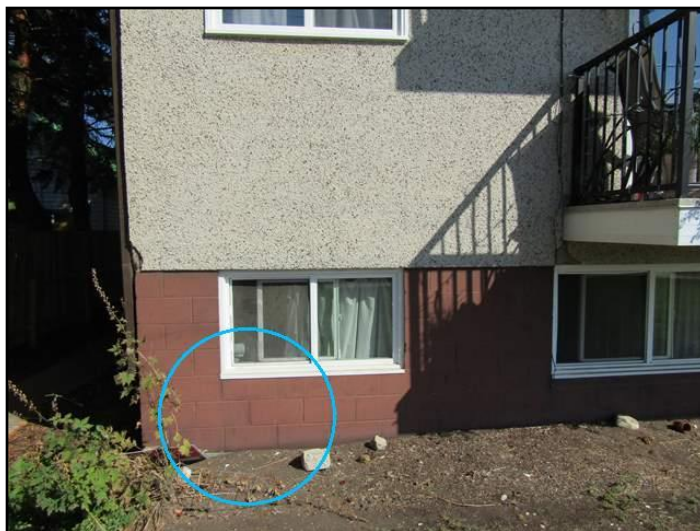
Step Crack
