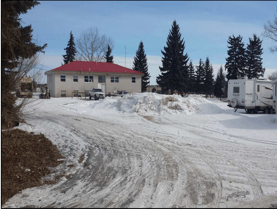
Photograph 3: Looking northeast across the back alley at the yard of the Property which featured a stockpile of cleared snow from the parking area at the time of the inspection (March 5, 2015).
