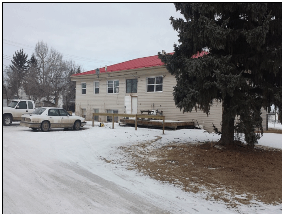
Photograph 2: Looking north at the back entrance of the apartment building and the parking stall area (March 5, 2015).
