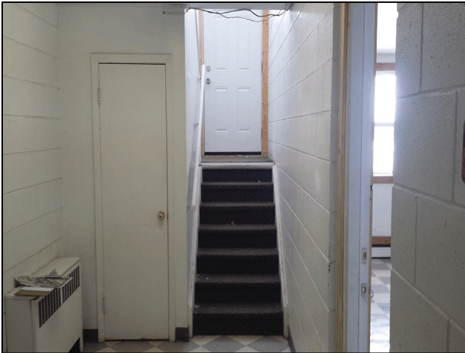
Photograph 4: Showing the lower level hallway of the building, with vinyl tile flooring, painted concrete block finishes and baseboard area heater (March 5, 2015).
