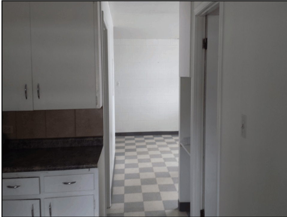
Photograph 5: Looking at the kitchen and living room of a rental unit in the building. Showing wood cabinets, laminate counter and ceramic tile finishes in the kitchen, and painted drywall and vinyl flooring throughout the rental unit (March 5, 2015).
