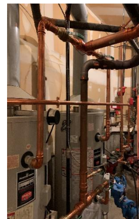
Figure 1 - DHW Tanks
