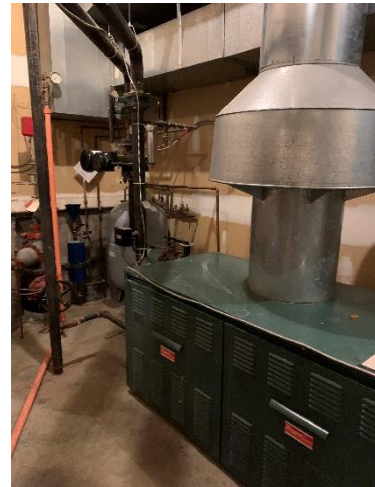
Figure 3 - Hydronic Boiler
