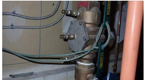
Cross Connection Control Devices
