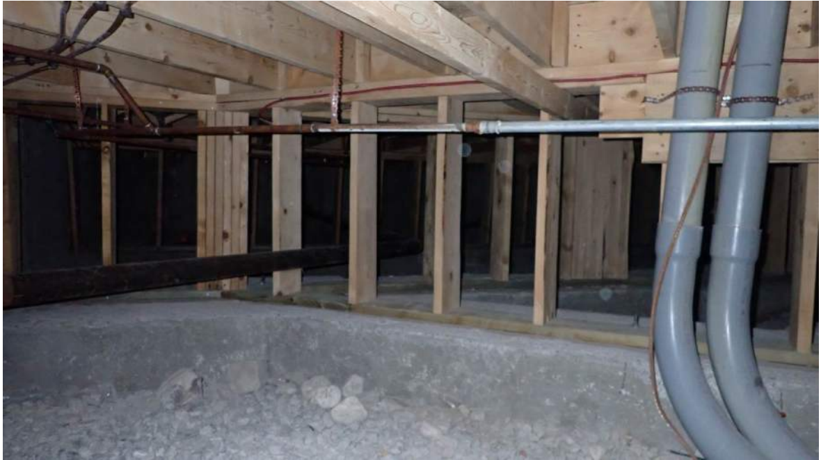
Photo 3 Building Foundation Crawl Space
