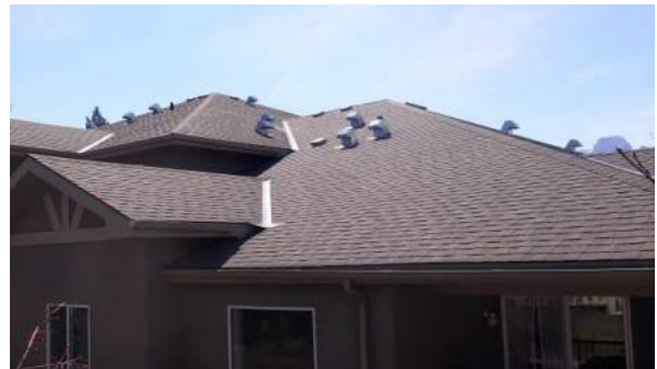
Sloped Shingle Roofing
