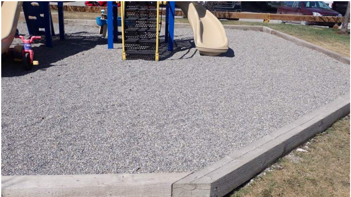
Photo 6 Playground Play Surface and Wood Curb
