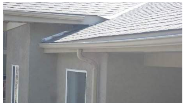
Eavestroughs/Downspouts/ Metal Works
