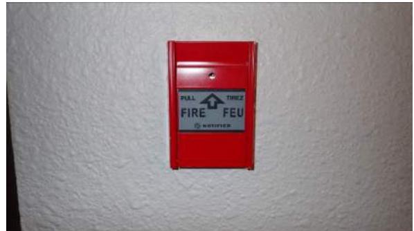
Signal Devices/Pull Stations
